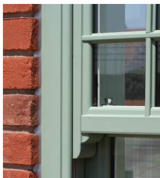
Run through sash horns
